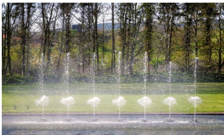
Efekt podbijania – Pop-Jet Effect – H_{\max} = 3,0\text{m}
